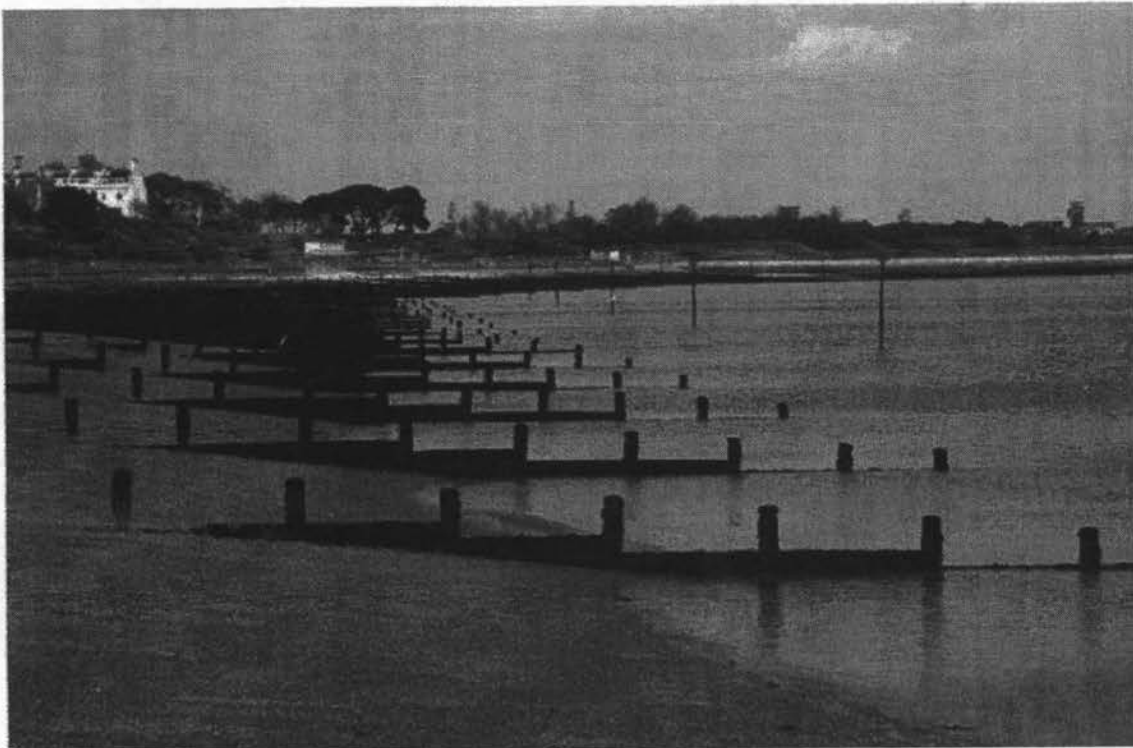
Photograph A for Question 3 Groynes along a coastline
