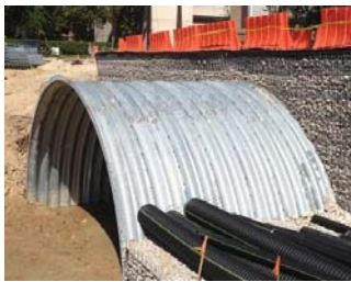
Diagram 1: Low-profile arch culvert
